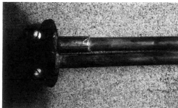
Sleeve in place after application of epoxy.
