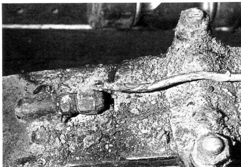
Figure 2: Even under the gaiter, you may find dirt or a broken Bijur line. No wonder these springs required overhaul.
